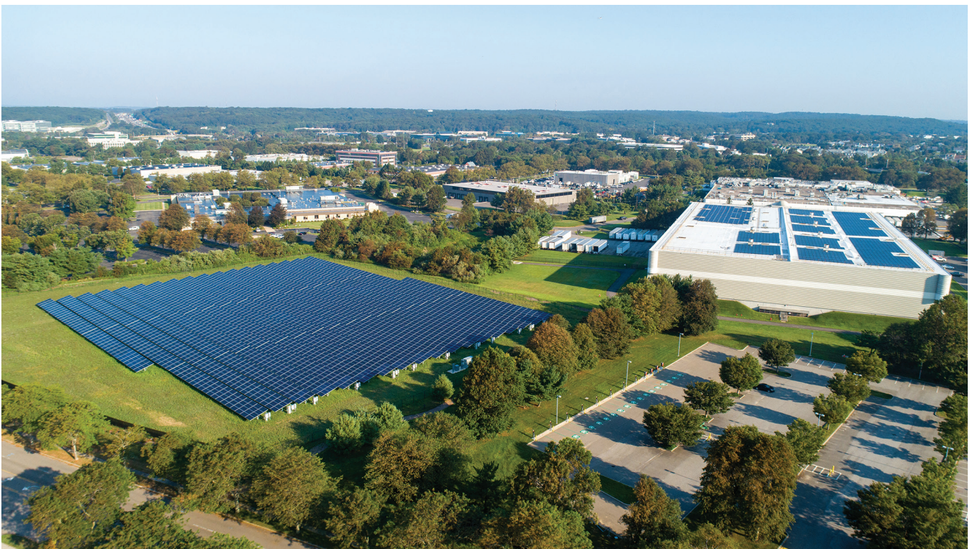
As part of their global citizenship and sustainability efforts, Estee Lauder Companies installed 2 MW of rooftop and ground mounted solar at their campus in Melville, NY. The array provides 100% of the electricity for their office. © EmPower Solar
