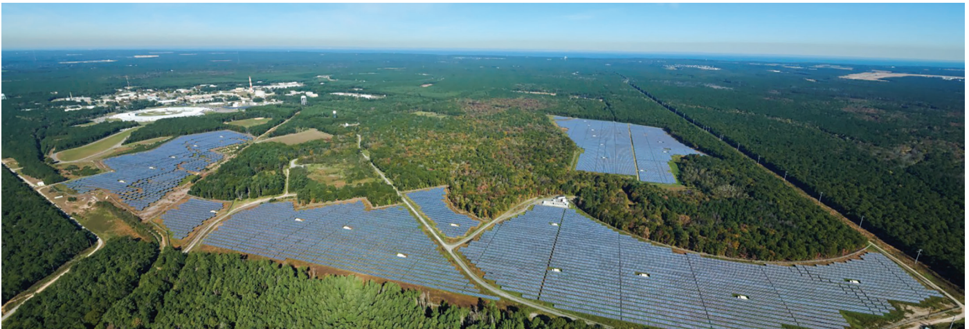
Long Island Solar Farm at Brookhaven National Laboratory © Long Island Power Authority
