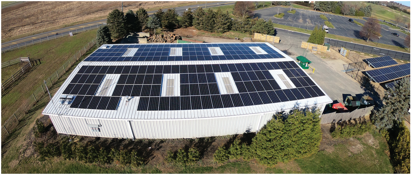
Rooftop and ground-mounted solar arrays at the Long Island National Golf Club in Riverhead © SUNation Solar Systems
