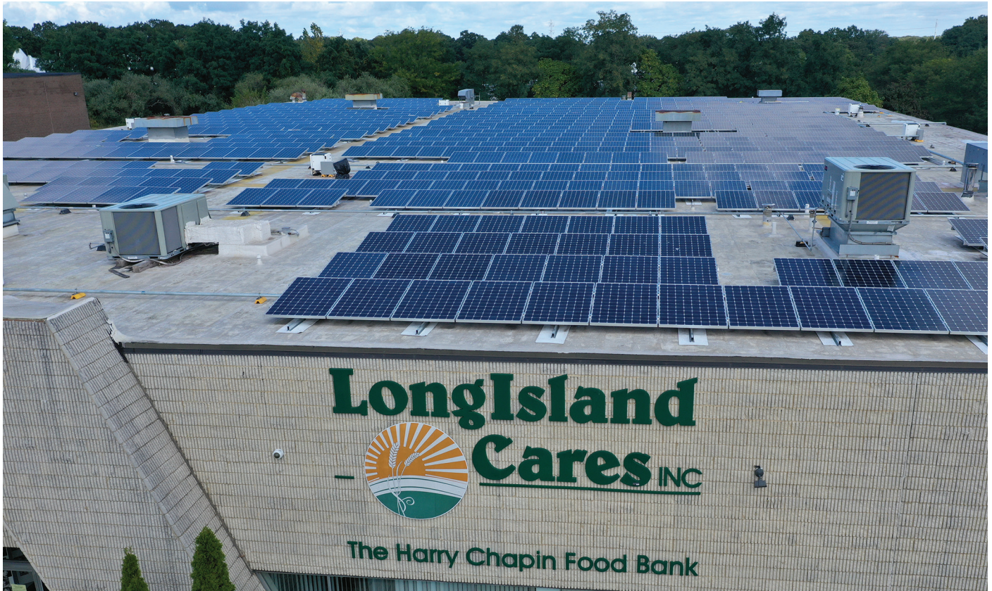
Long Island Cares installed solar on the roof of its headquarters—the Harry Chapin Food Bank located in the Long Island Innovation Park at Hauppauge. This community solar installation provides renewable energy to approximately 50 households experiencing hardship and food insecurity and is part of a larger strategy by the Hauppauge Industrial Association’s Solar Task Force to transition the business park to renewable energy. © SUNation Solar Systems
